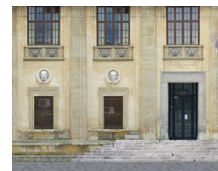
Facade orthomosaic GeoTiff (.tif)
